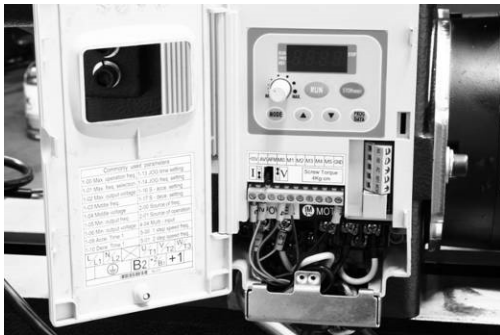
VFD with cover open
